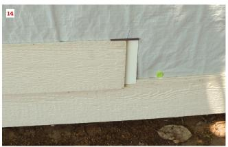
with a chalk line or a straightedge. These marks represent the *bottom* edge of each course and will be impossible to see as the siding is installed. So after the reference lines are drawn or snapped, I transfer them onto the edge of the trim where they can be read as the siding is installed.
